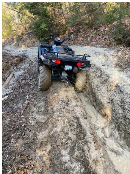
The heavily eroded section of the Community Centre By-Pass Track in the spring of 2021. Even Reg Smart's ATV got stuck in the muck.
